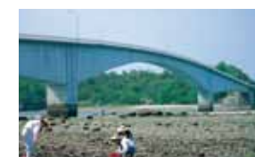
Third Bridge (Nakanohashi Bridge) [B-7]
