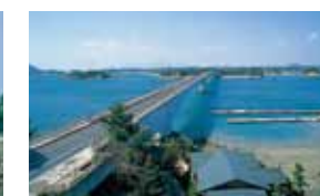
Fourth Bridge (Maeshima Bridge) [B-7]
