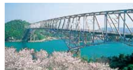
First Bridge (Tenmon Bridge) [A-7]
