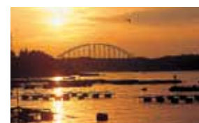
Second Bridge (Oyano Bridge) [B-7]
